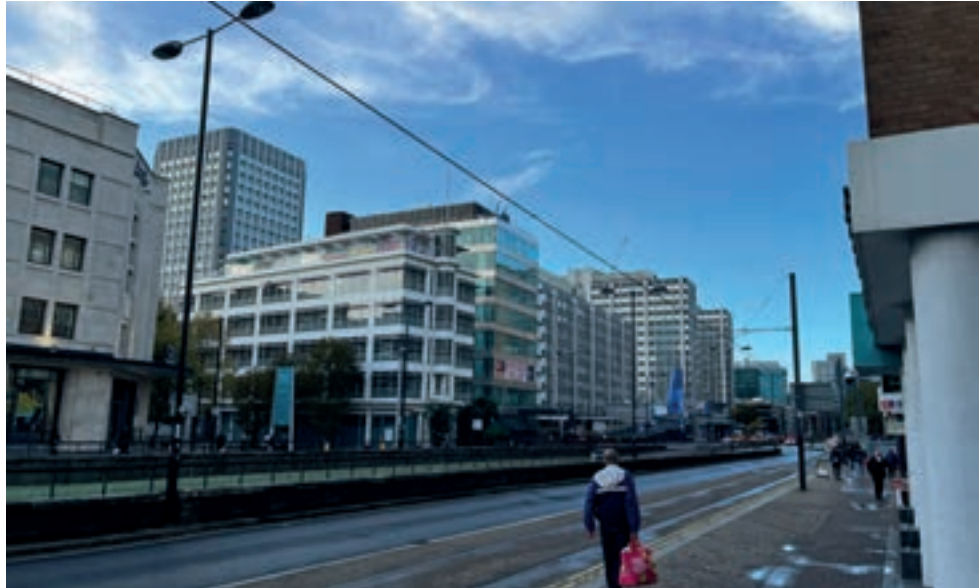
Fig 70 Wellesley Rd dominated by road infrastructure
