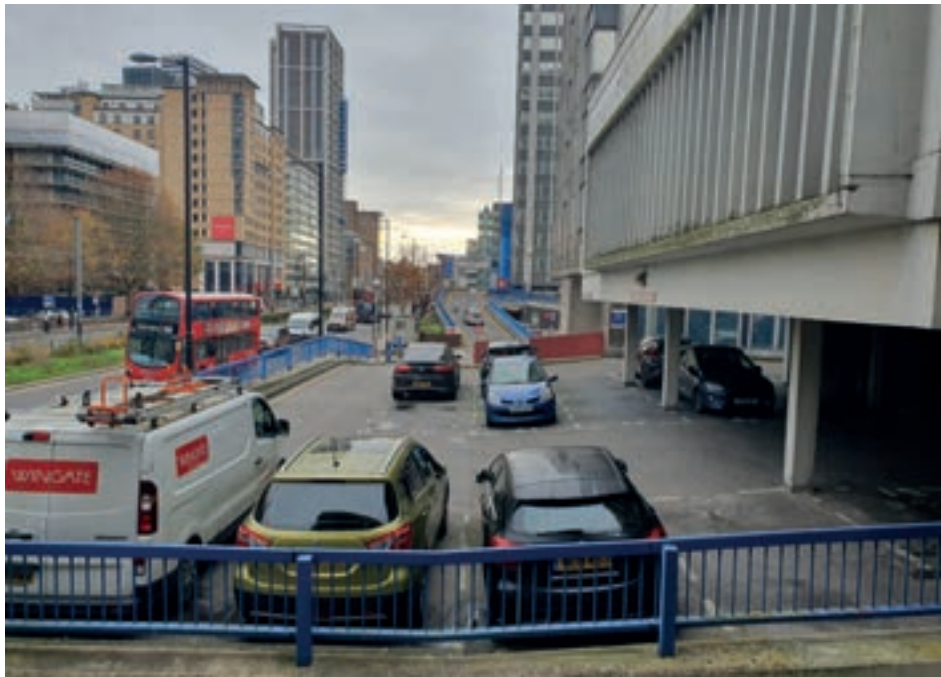
Fig 41 Wellesley Road looking south - access to the various existing car parking areas is via a complex set of ramps
