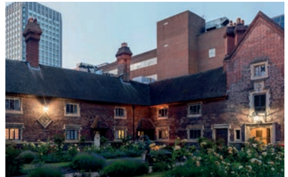
Fig 54 Today: View north east across the private Almshouses courtyard
