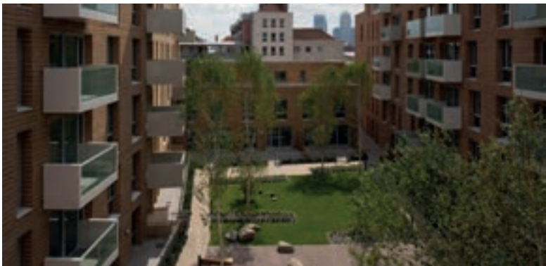
Fig 88 Private courtyard: St Andrews, Bow
