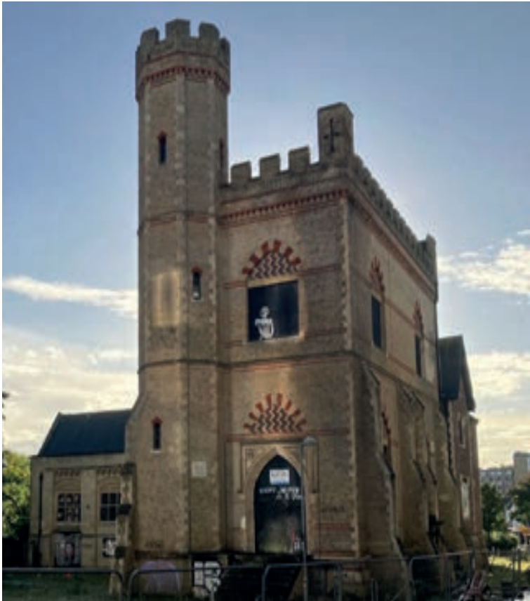
Fig 25 The Surrey Street Pumping Station
