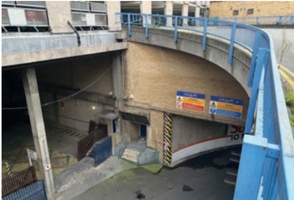
Fig 42 Exit ramp from the Whitgift Centre car park via Poplar Walk
