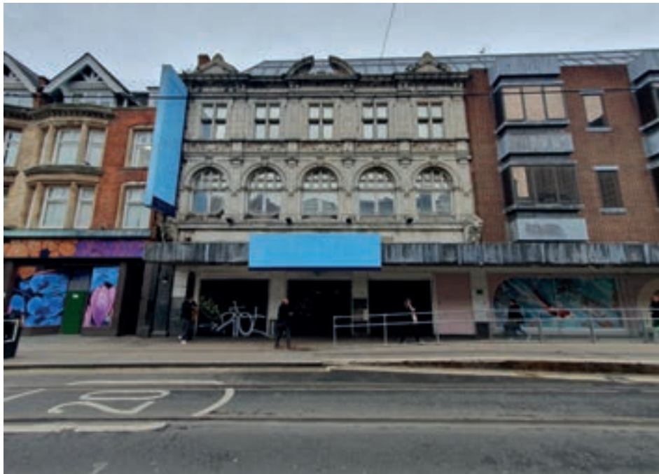
Fig 43 The George Street entrance to the former Alders Store
