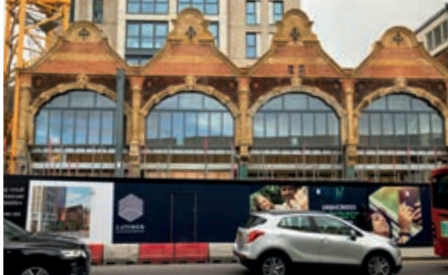
Fig 27 Station Road mixed use re-development
