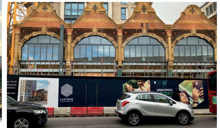
Station Road mixed use re-development
