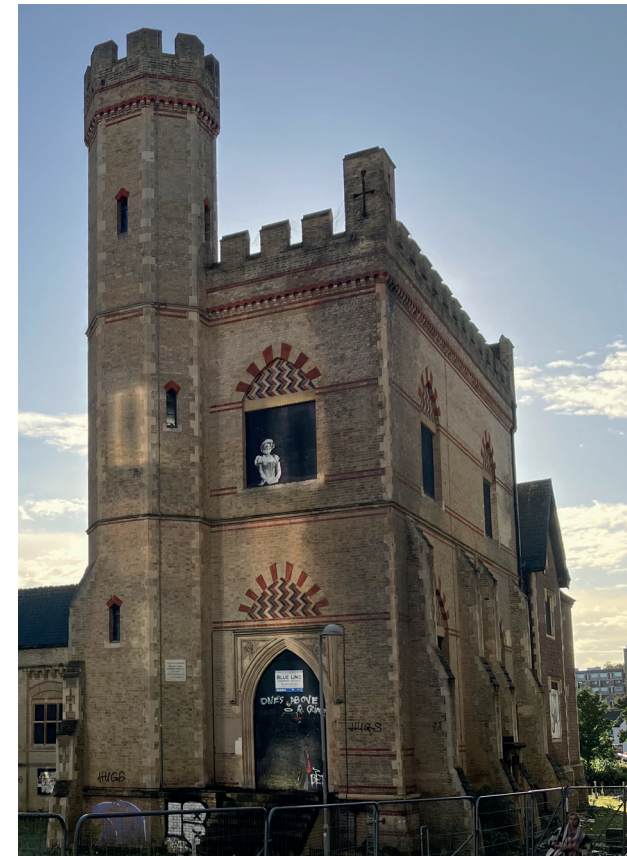
The Surrey Street Pumping Station
