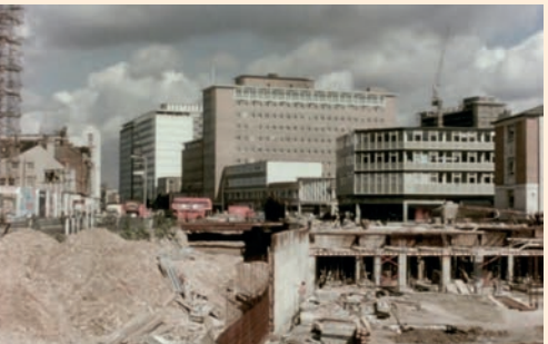
Redevelopment underway in Croydon, c.1960s (Source: BFI)
